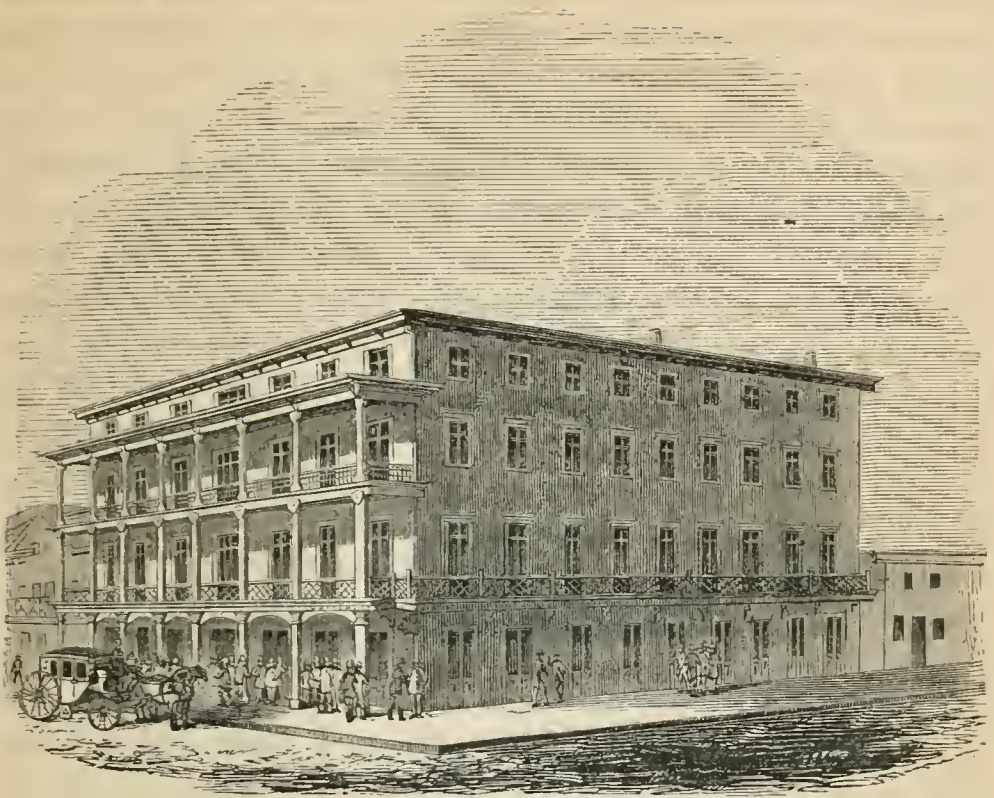
Oriental Hotel, corner of Battery and Bush streets.
